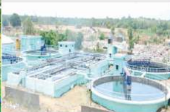
Sewage Treatment Plant
