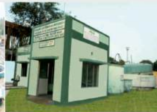
Bio Gas Waste to energy
